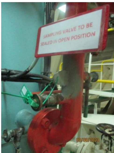
Figure 6 – sample line valve to 15ppm bilge alarm open with signage fitted.
