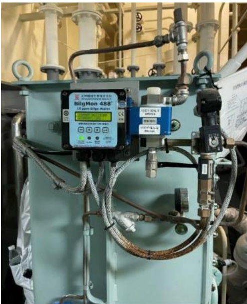
Figure 4 - a flow sensor and alarm fitted to the 15ppm bilge alarm sample line.
