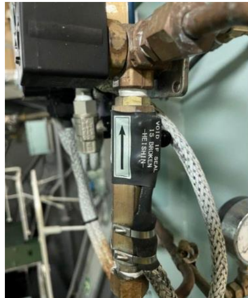
Figure 5 – a detailed view of a flow sensor and alarm fitted to the 15ppm bilge alarm sample line.
