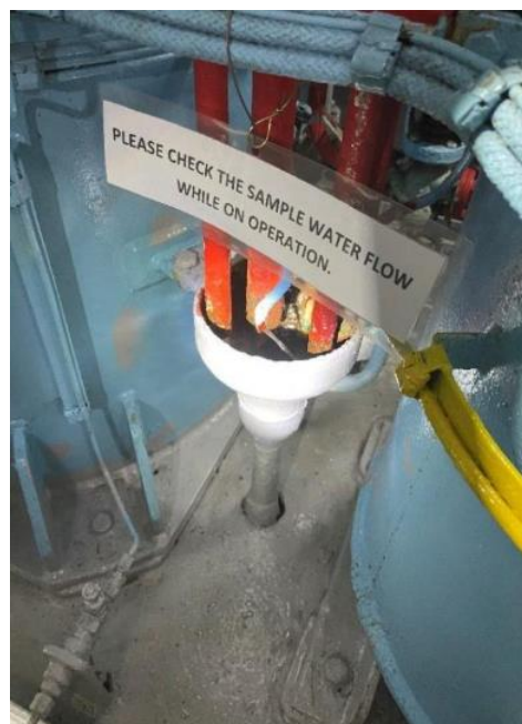
Figure 7 – a verification of flow of sample water from sealed open with signage fitted.
