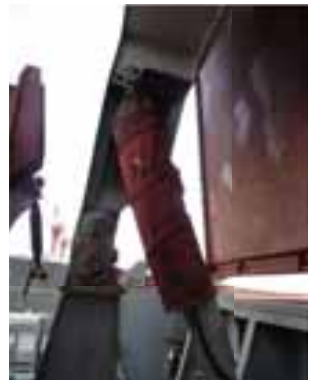
Photograph 21 Protective sleeve for cylinders
