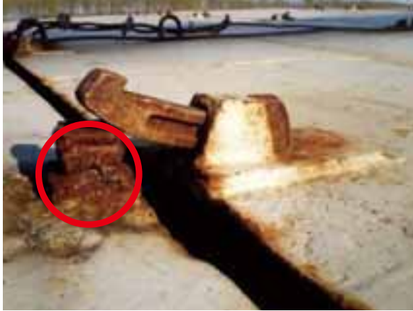
Photograph 17 "Banana shaped" cross wedge with striker plate built up
