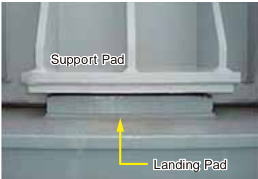
Photograph 10 Support Pad & Landing Pad
