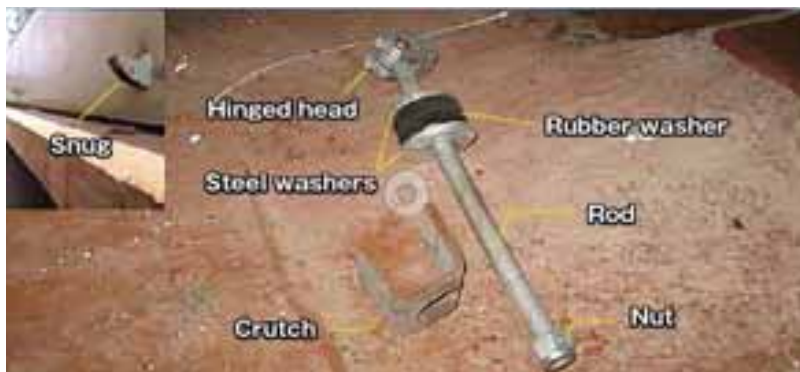
Photograph 16 Quick acting cleat parts
