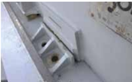
Photograph 15 Panel stopper arrangement
