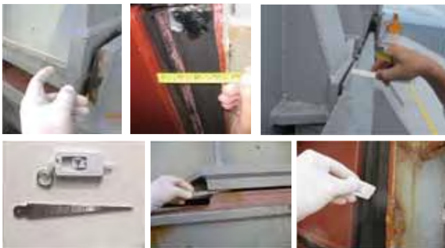
Photograph 3 Using feeler gauges, yardsticks and depth gauges during an inspection
