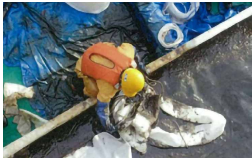
Photograph 24: Recovery Work Using Oil Adsorbent
