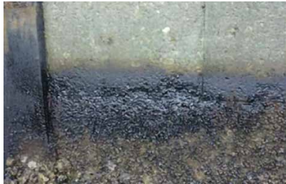
Photograph 27: Quay Wall Spoilage
