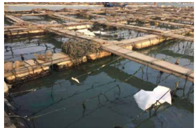
Photograph 11: Damage to Fishing Facilities
