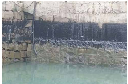
Photograph 16: Fuel Oil Washed Ashore against Seawall
