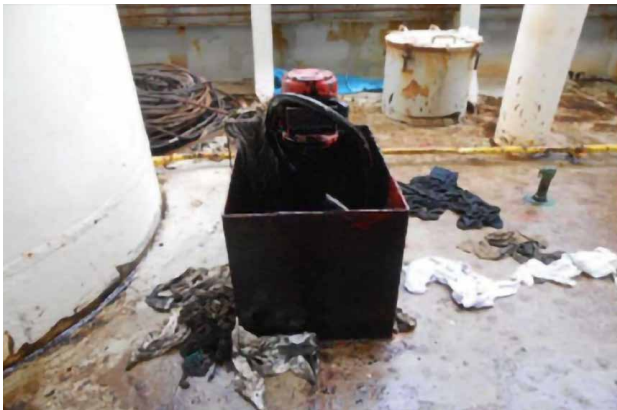
Photograph 17: No.2 C FO Tank Air Vent.
