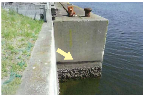
Photograph 22: Seawall Spoilage by Oil Washed Ashore
