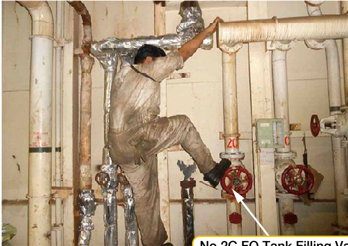
No.2C FO Tank Filling Valve
