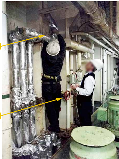
Photograph 18: Insulation Installation
