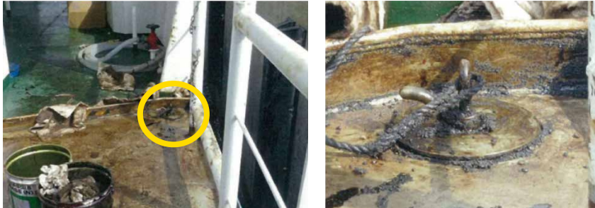
Photograph 23: Seawall Scupper Spoilage Caused by Oil Leakage
