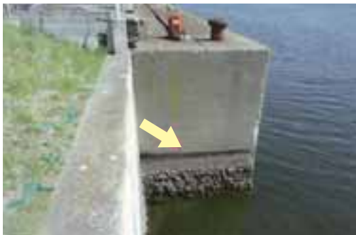
Photograph 22: Seawall Spoilage by Oil Washed Ashore
