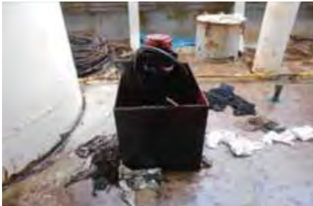
Photograph 17: No.2 C FO Tank Air Vent.
