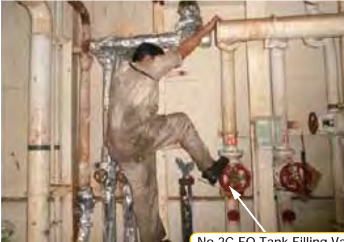
Photograph 19: Reason Why No.2C FO Tank Filling Valve Opened
