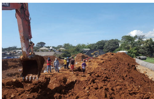
Sampling nickel ore by excavator
