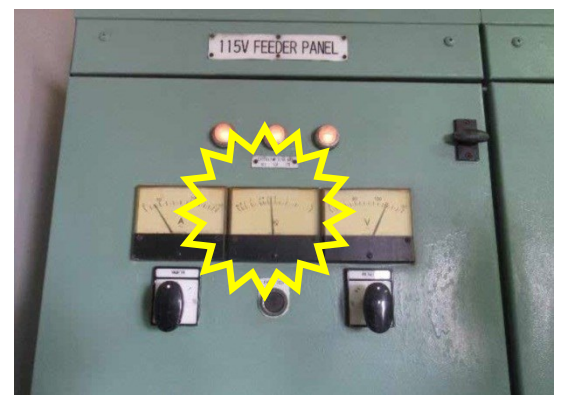
Poor insulation of electric circuit
