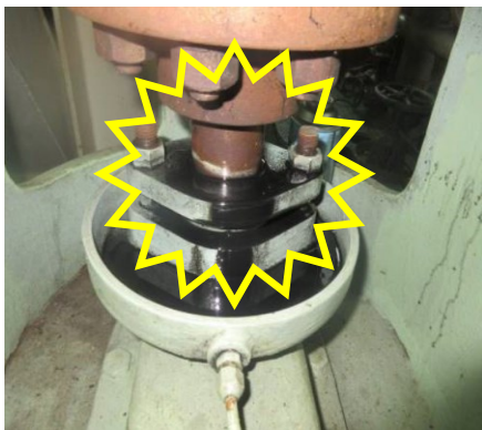
Oil leakage due to deterioration of gland-packing
