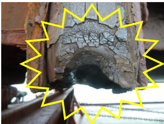
Rubber gasket on hatch cover, broken and deformed due to compression and hardening.
