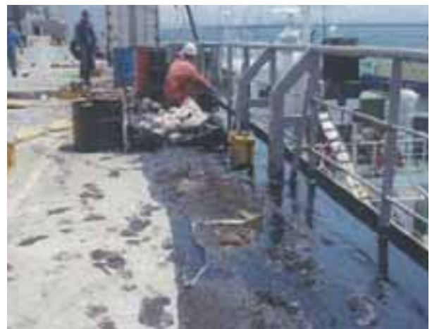
Reference Picture 40 Port side of upper deck
