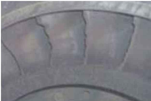
c) Damaged nozzle ring (Over run) Damage leading to speed reduction in fiscal year 2014 / reference *4
