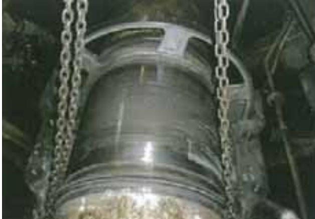
a) Burn-out Intermediate shaft bearing (Over-heated) Damage requiring towing in fiscal year 2013 / reference*8
