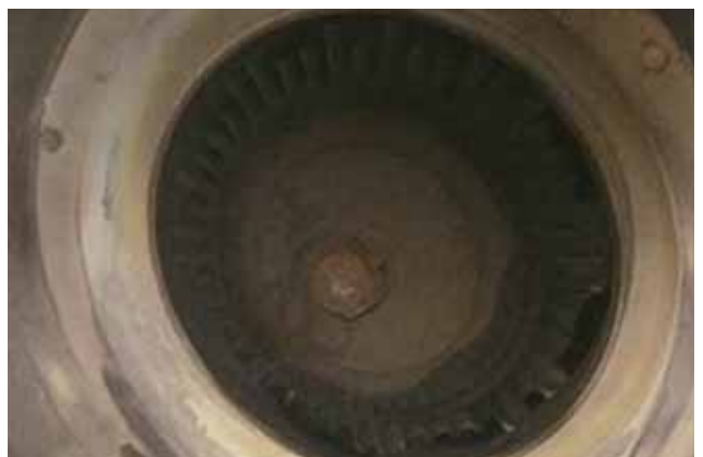
f) Broken turbine blade Damage leading to speed reduction in fiscal year 2013/ reference *8
