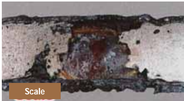
Figure 38 Broken hole due to scales / reference *12
