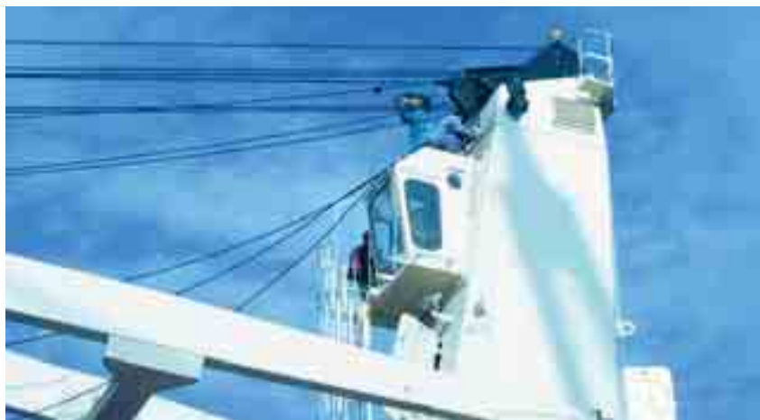
Photo 2 Maintenance on-going at the top of a crane
