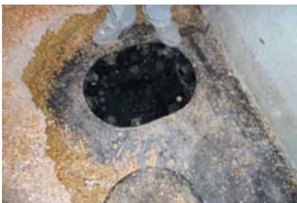
Fig.11 Lime wash remaining on a bulkhead after the discharge of a sulfur cargo. The scratch marks at the base of the bulkhead are from the o -loading operation.
