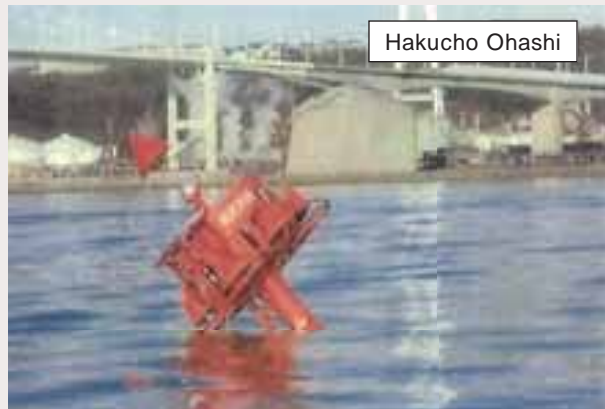
Photograph 67 Damaged state of No.2 light beacon
