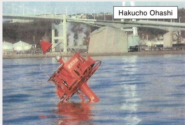
Photograph 67 Damaged state of No.2 light beacon
