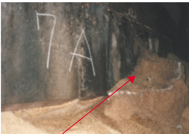
Showing heavily caked and discoloured cargo along bulkhead plates between the engine room and the aftermost hold
