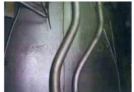
Figure36 Upper boiler casing (Paint swelling)
