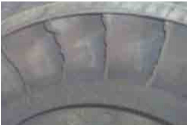
c) Damaged nozzle ring (Over run) Damage leading to speed reduction in fiscal year 2014 / reference *4
