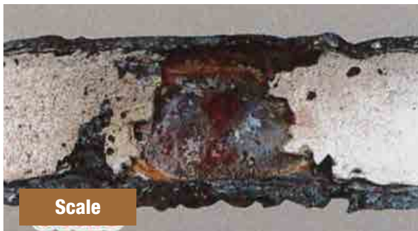
Figure 38 Broken hole due to scales / reference *12
