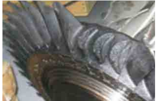
b) Broken turbine blade Damage leading to speed reduction in fiscal year 2014 / reference *4
