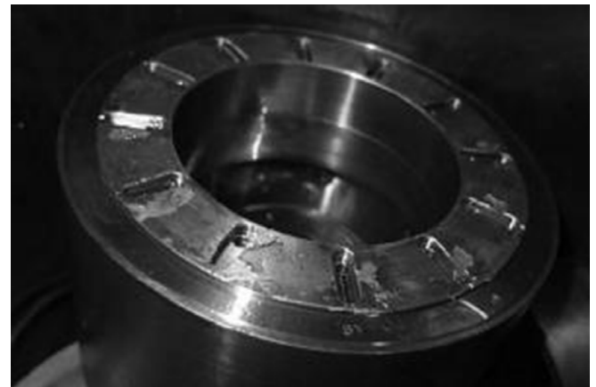
Figure 19 Thrust bearing with metal peeled off / reference*7
