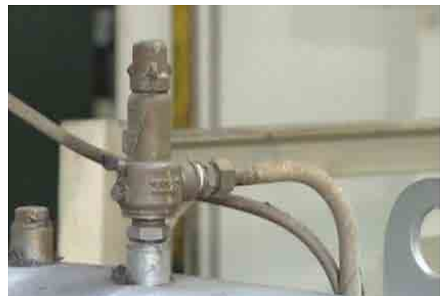
Figure 96 Leaking safety valve of fuel oil heater
