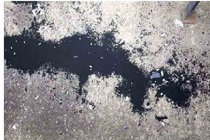
Figure 62 Soot on working passage of factory
