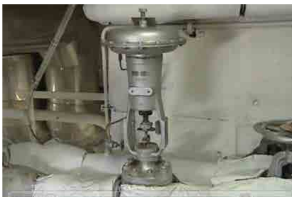
Figure 97 Damage of diaphragm on control valve
