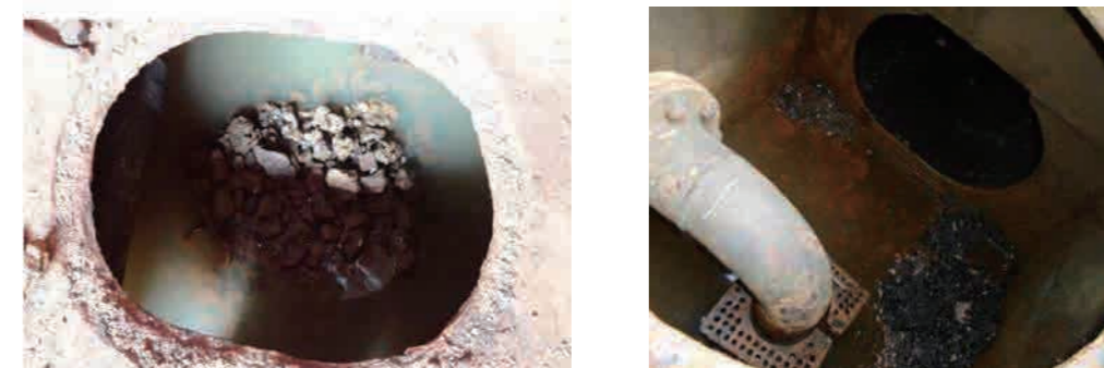
Note: Last cargo from the previous voyage remaining in the bilge well and blocking discharge of bilge water.
