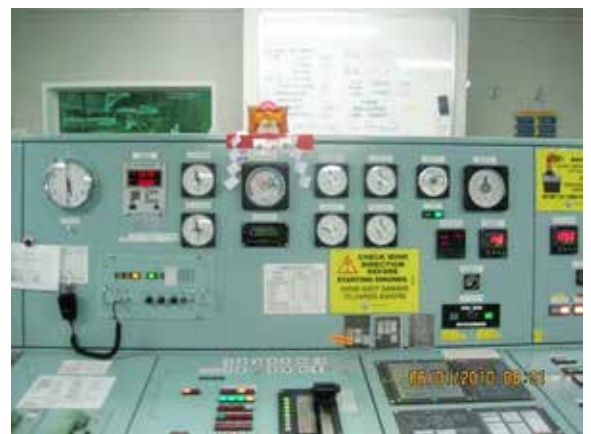
Engine Control Room Console
