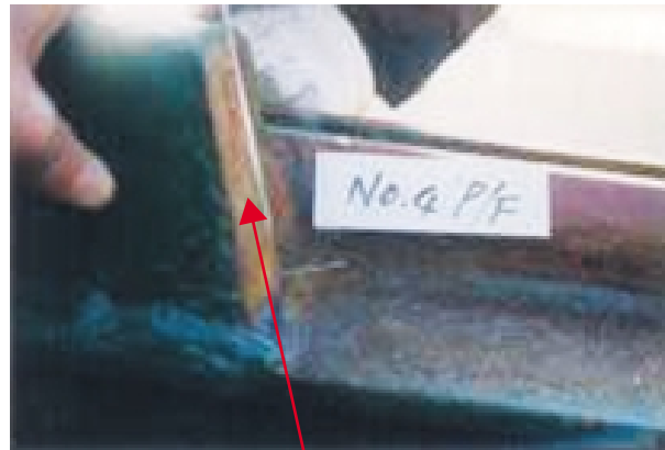
Showing heavy wear down at the contact face of the rest
