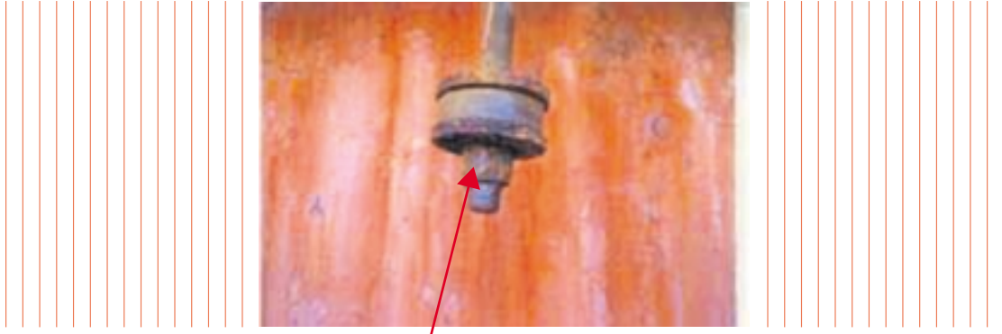
Bolt に錆付いたAdjusting nut
