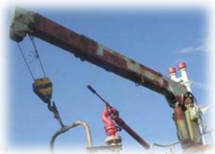
SWL (Safety working load) not marked on lifting gear or marked but unclear
