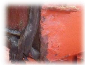
Defective rubber gaskets on hatch covers
