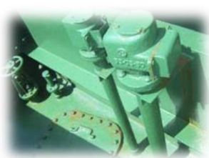
Names of related tanks for sounding pipes, air vent pipes not marked
