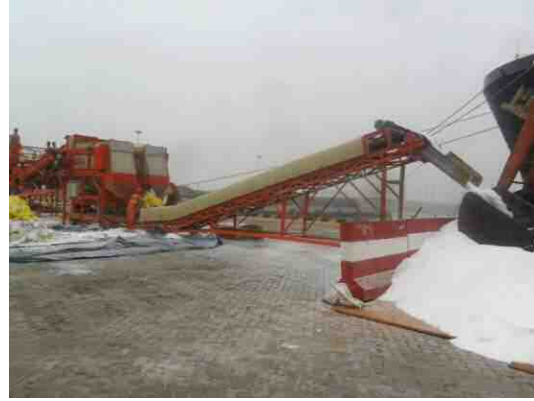
The fertilizer is transferred to the storage yard for crushing by grinder
